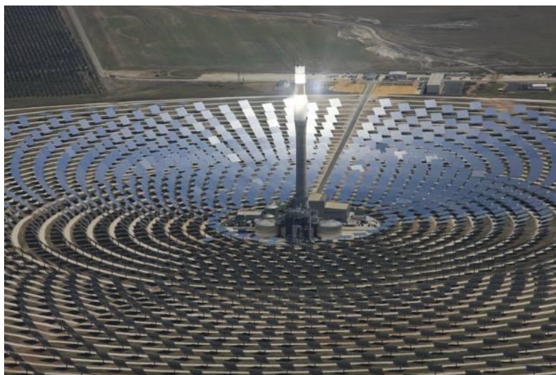
Figure 2-2: Central Receiver system, Spain. ( Gemasolar plant, owned by Torresol Energy (c) Torresol Energy)
