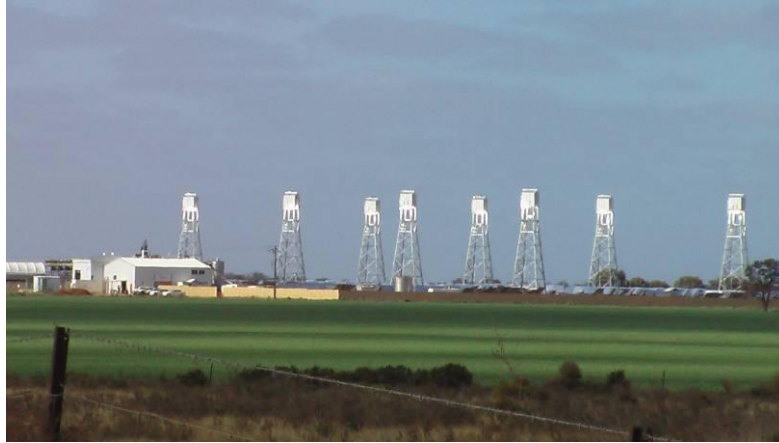
Figure 3-13: Multi tower, graphite energy storage demonstration at Lake Cargelligo, NSW (picture K Lovegrove).
