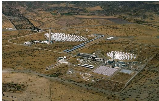
Figure 2-10: Plataforma Solar de Almería site (picture www.psa.es/webeng/index.php ).
