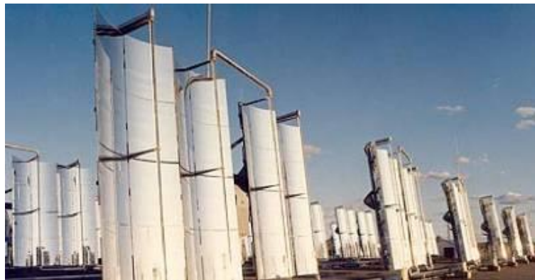
Figure 3-6: Meekatharra Collectors, (WA World of Energy).
